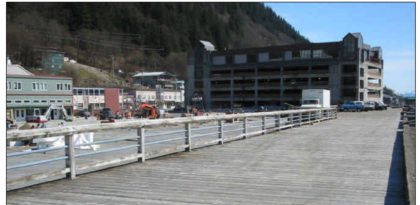
View of the Steamship Wharf and the Juneau Public Library/Parking Garage (Area C)
